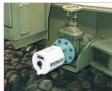
Horizontally on the drain valve
