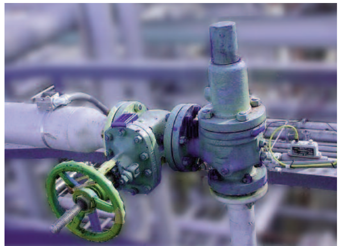
Figure 1: Typical Pressure Relief Valve
